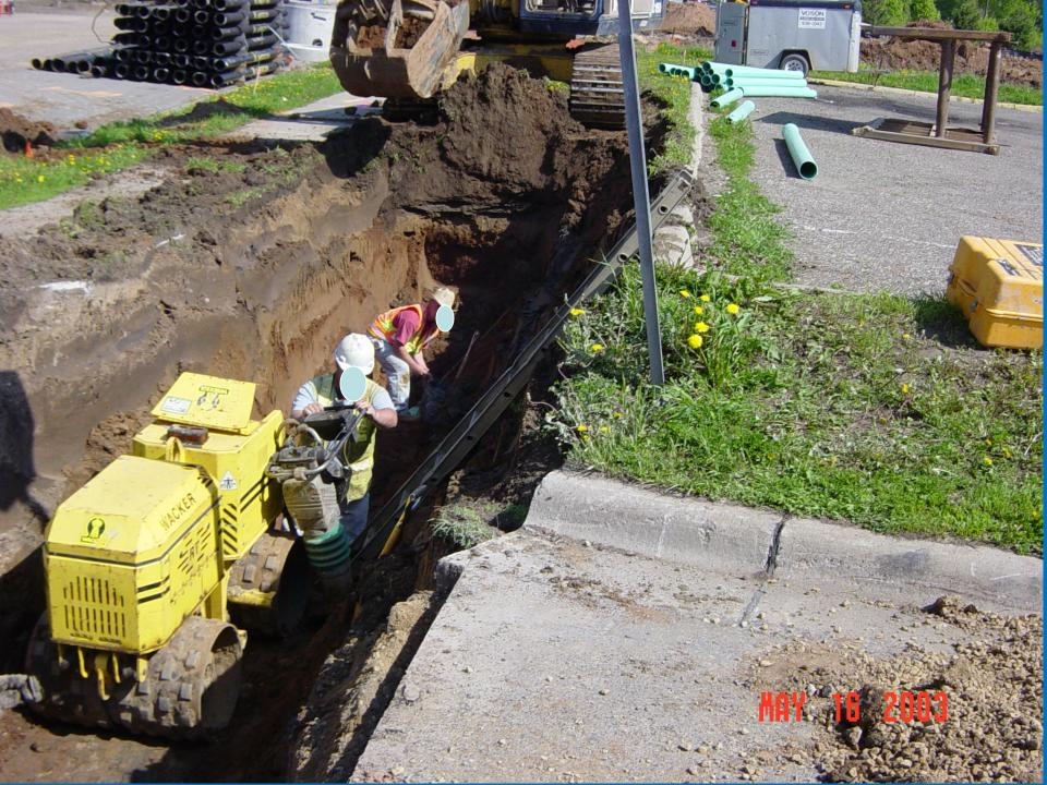
Mobile equipment warning systems When an equipment operator does not have a clear and direct view of the edge of the excavation:
